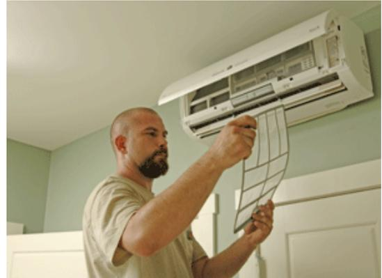
**3. Clean Indoor Unit Coils** Check to be sure that the evaporator coils are clean. Though indoor air handler coils are amply protected by the various levels of filtration, it's good to examine coil cleanliness each year. Coils usually require cleaning on a bi-annual basis. Typically, evaporator coil cleaning entails:
